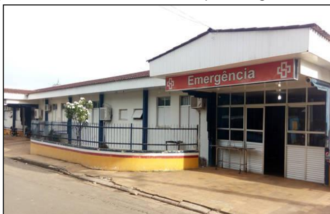
Figura 2 – Vista Externa do Hospital Regional de Tefé
