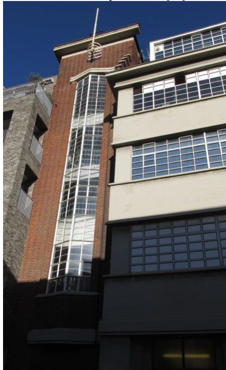
Figura 30 – Edifício British Museum Department of Africa, Oceania and Americas
